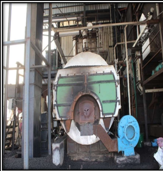
Machinery name: Coal fire boiler Location in plant: Hot air generator Capacity: 2000KGS Use: Boiler to Provide Steam
