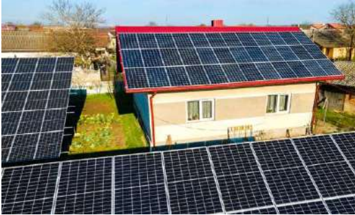
Rajasthan State domestic Rooftop under RREC scheme 2 MW
